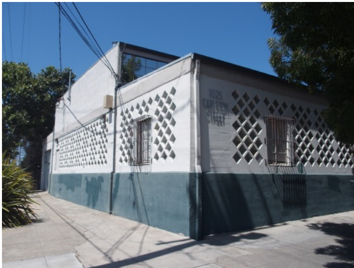
Concrete grid form building
