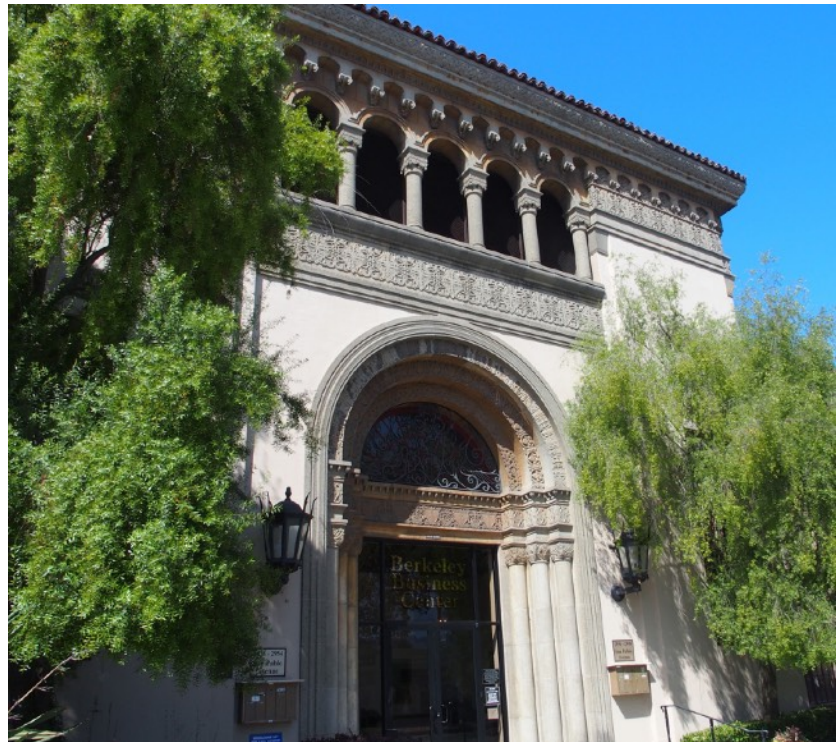
Entry to former Heinz building
