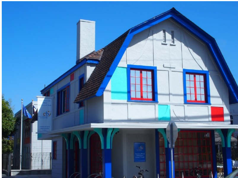
Ecole Bilingue Historic Building
